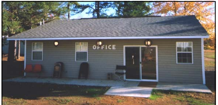
AFTER Front of Office Building
