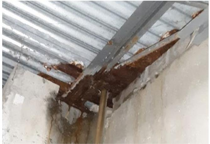
Photo: rust at underside of decking at drain lines.
