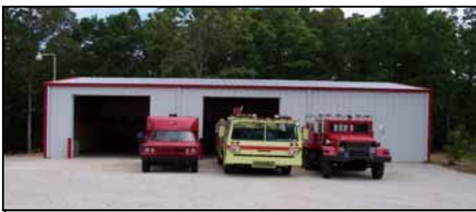
Ruthie Mountain Volunteer Fire Department's new fire station built with funds from the Rural Services Block Grant Program.
